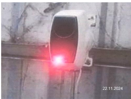
Smoke Beam Detector
